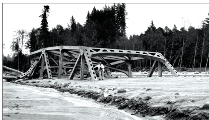
Figure 3. Washington State Highway 504 steel bridge structure carried about 0.5 kilometers (0.25 miles) downstream and partly buried by the May 18, 1980, mudflow from Mount St. Helens. Photograph by R.L. Schuster, U.S. Geological Survey.
