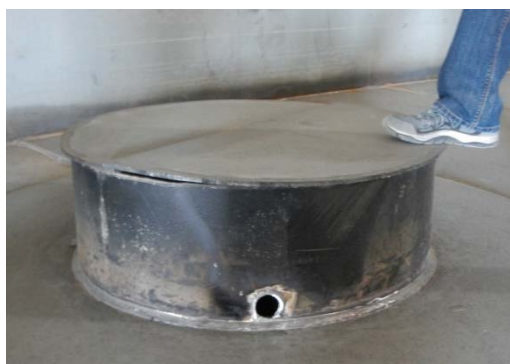
Figure 28. Raised inlet/outlet line (silt ring) installed by Bohannon Huston in an 11,000 m 3 (3 million gallon) water tank installed in Albuquerque, NM. The cover on top of the ring would be removed during normal operation. The small hole on the side allows for complete tank drainage.
